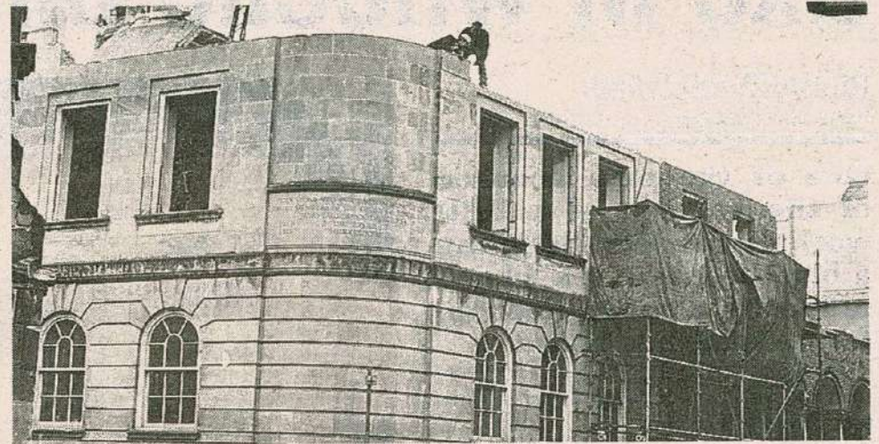
The old Shirehall in The Square, Shrewsbury, being demolished in 1971
